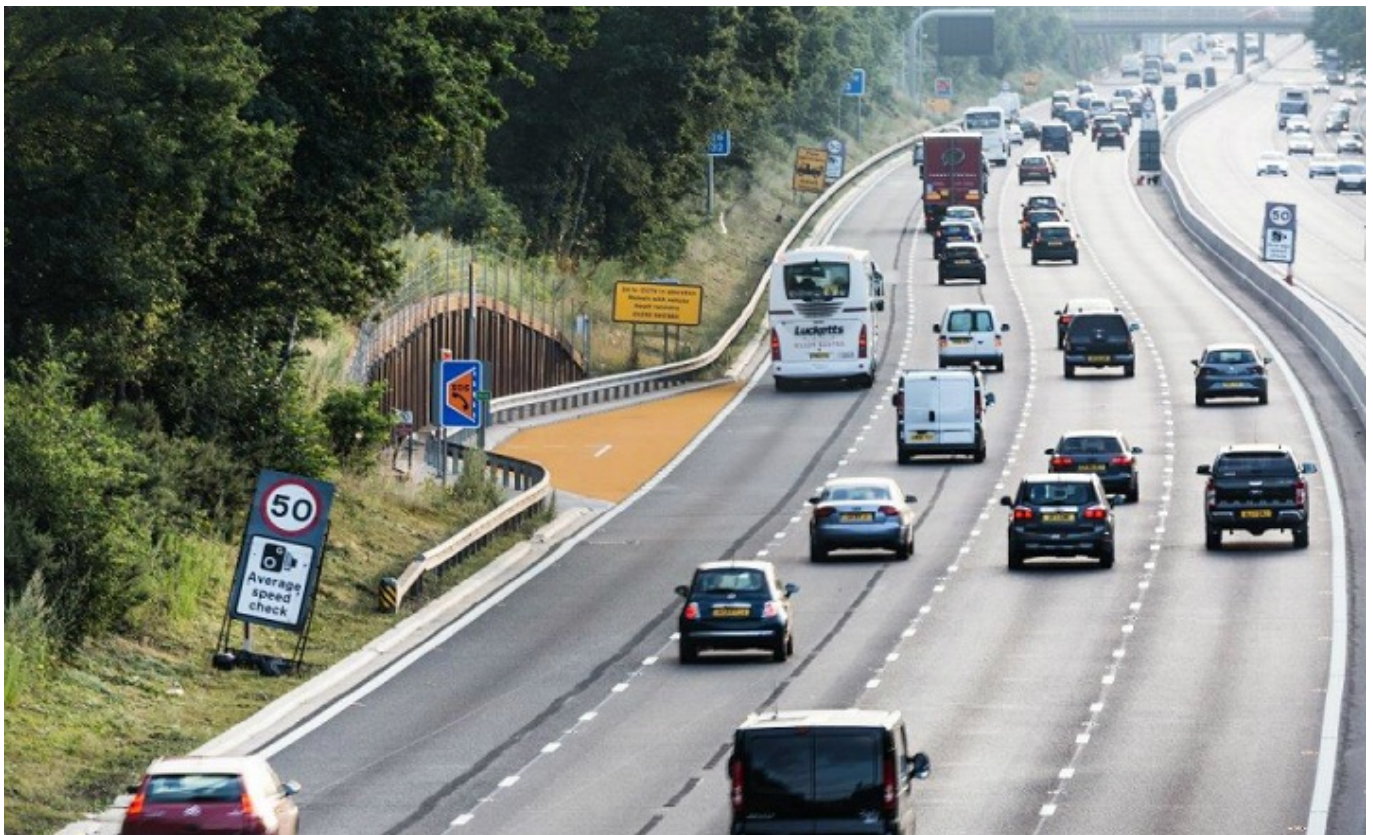
Photograph by Highways England.
