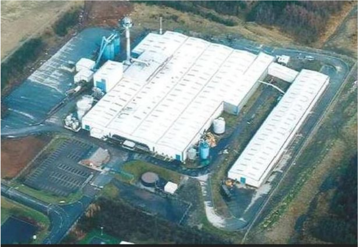
TVR factory aerial view.
